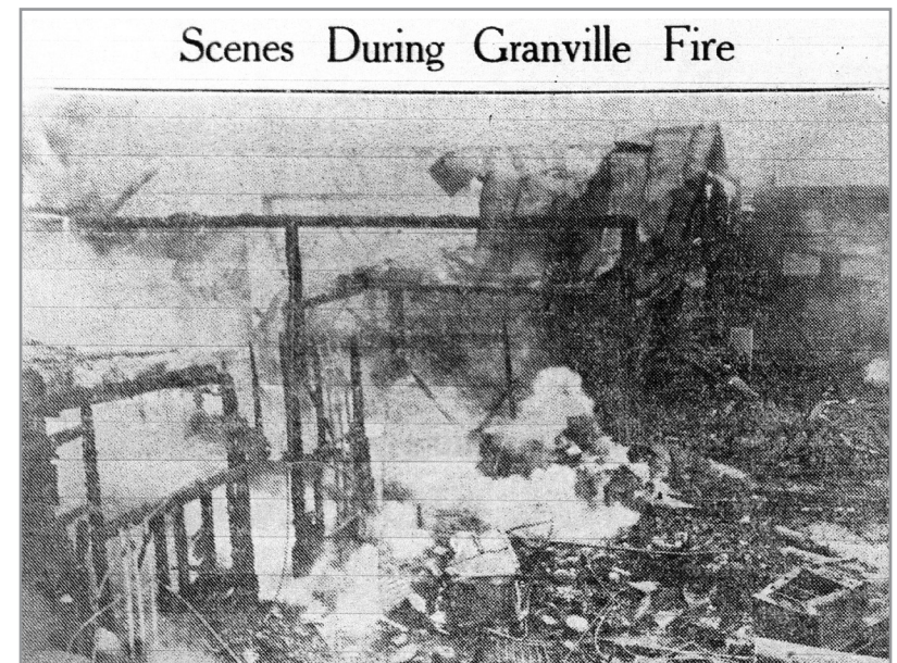
This faded picture from the Granville Times depicts the extent of the destruction of the 1927 fire that obliterated most of the shops on the south side of the 100 block of East Broadway. Although it's hard to make out, you can see the remnants of buildings lost in the conflagration.
